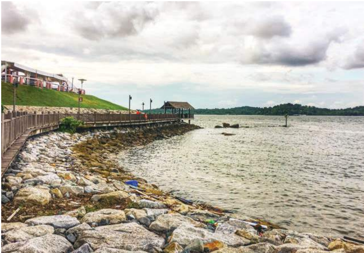
Coastal areas can be vulnerable to rising sea levels
