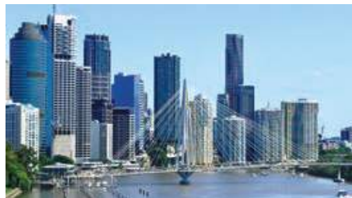
The Kangaroo Point Bridge, a project under the Brisbane City Plan, opened in December 2024 with dedicated paths for pedestrians and cyclists 439
