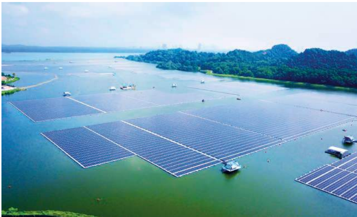
The Sembcorp Tengeh Floating Solar Farm is one of the world's largest inland floating solar farms
