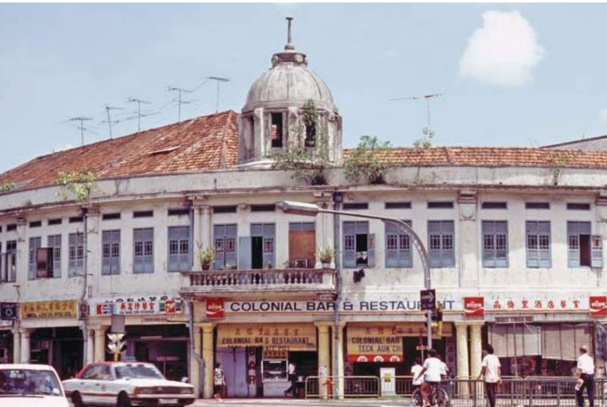
Built in 1924, the Ellison Building is a colonial-style structure situated at the junction of Selegie Road and the Mount Sophia Conservation Area G P Reichelt Collection, courtesy of National Archives of Singapore
