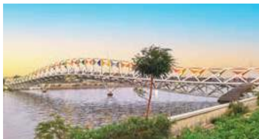
The Atal Pedestrian Bridge was built across the Sabarmati Riverfront
