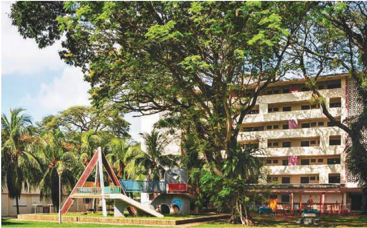
HDB blocks in the Dakota Crescent housing estate were identified for the Selective En bloc Redevelopment Scheme in 2014
