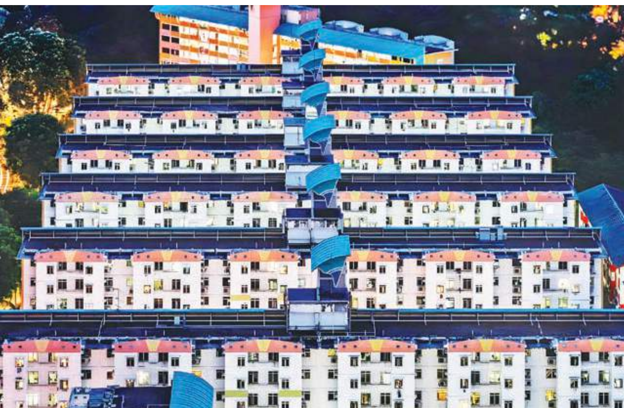
HDB blocks in the Tanglin Halt housing estate were identified for the Selective En bloc Redevelopment Scheme in 2014
