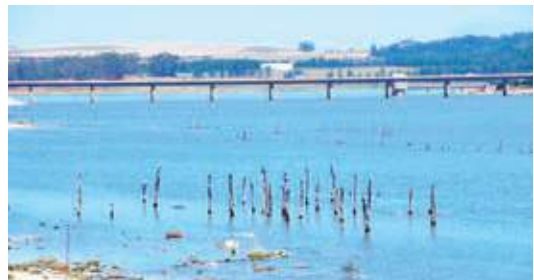
Theewaterskloof Dam in South Africa is one of the key dams supplying water to Cape Town 434
